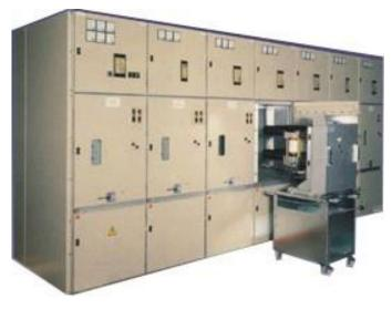
VCBs are the preferred choice at HV; absence of air and moisture in the arc-quenching medium (vacuum) results in zero contact erosion. They offer better service than SF<sub>6</sub>CBs, which suffer from problems of SF<sub>6</sub> gas leakage. The vacuum bottles used in VCBs are factory-sealed and have an operating life of up to 30,000 to 1,00,000 operations. Surge Arrestors are used with VCBs to suppress switching surges. Vacuum Contactors, a variant of VCBs are
